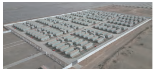
CNPC's Tarim Oilfield 600MMh Photovoltaic Power Generation Project
